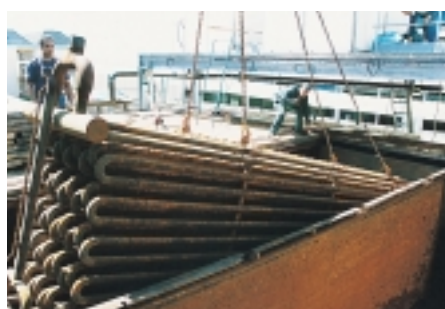
Removal of coils
